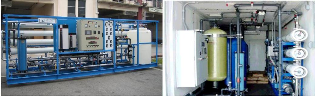
**Figure 2-28 Integrated SWRO installed in a customized 20' ISO shipping container**
